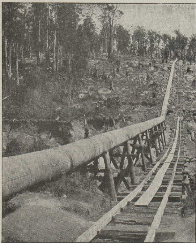
4—A Siphon Completed.
